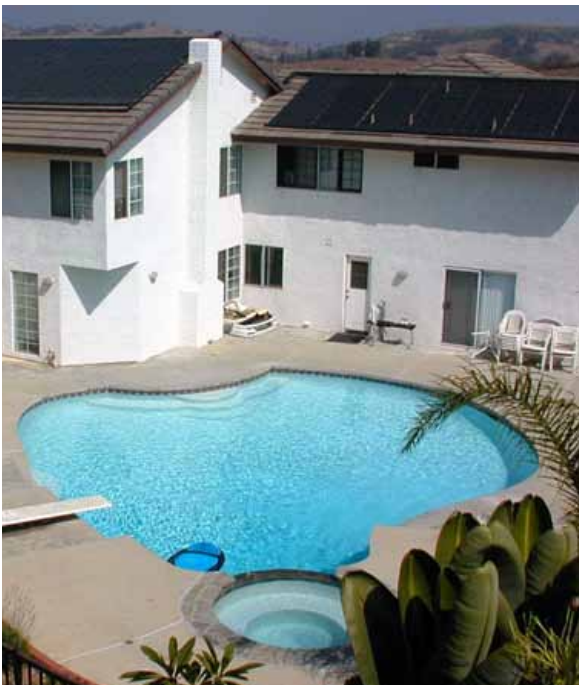
Solar heated pool in California
