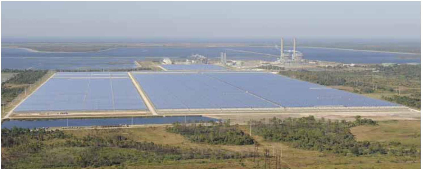
75-MW Martin Solar Plant near Indiantown, Florida
