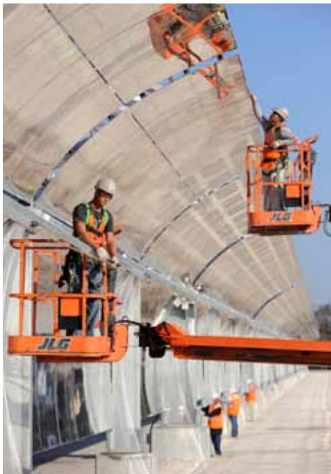
Construction of 75-MW Martin Solar Plant
