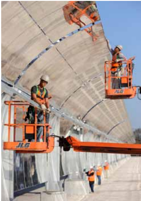
Construction of 75-MW Martin Solar Plant
