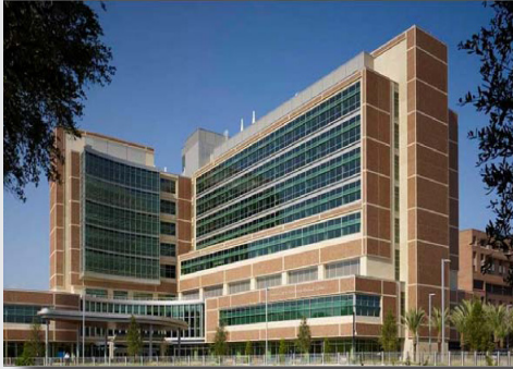
GRU owns and operates the microgrid at Shands Hospital in Gainesville, FL.
