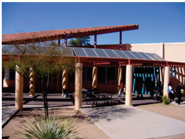
A 6 kW system at Doolen Middle School in Tucson, AZ. (Photo: Technicians for Sustainability)
