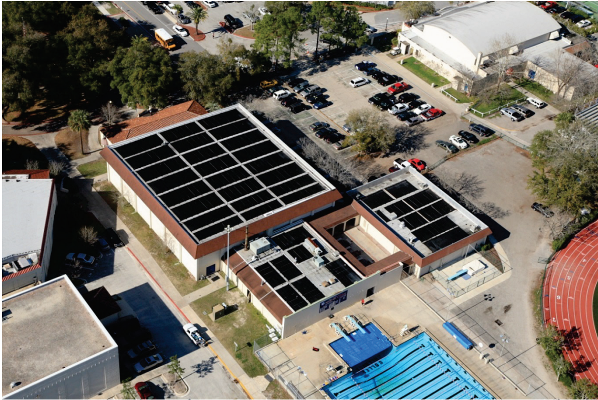
The Bolles School in Jacksonville, Florida has a 15 million BTU/day solar pool heating installation. (Photo: Solar Source)
