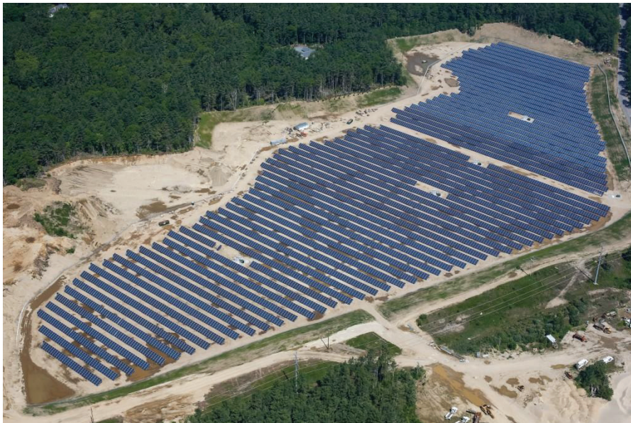
A 5,750 kW solar project in Plympton, MA, that powers Plymouth Public Schools. (Photo: Greg M. Cooper / Borrego Solar)
