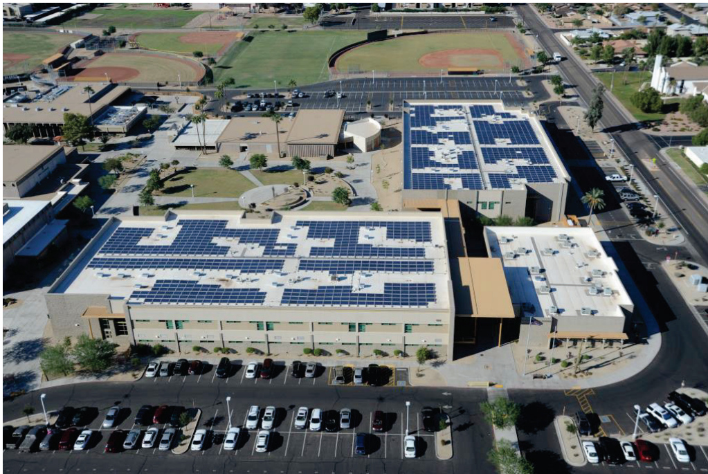
The Scottsdale Unified School District in Scottsdale, Arizona installed more than 2 MW of solar across four school sites to lock in years of future energy. (Photo: SolarCity)
