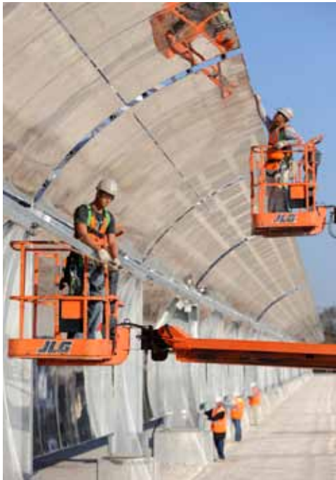
Construction of 75-MW Martin Solar Plant
