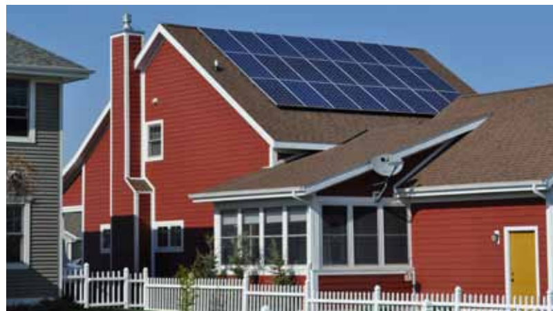
Residential photovoltaic installation in Plymouth, Wisconsin
