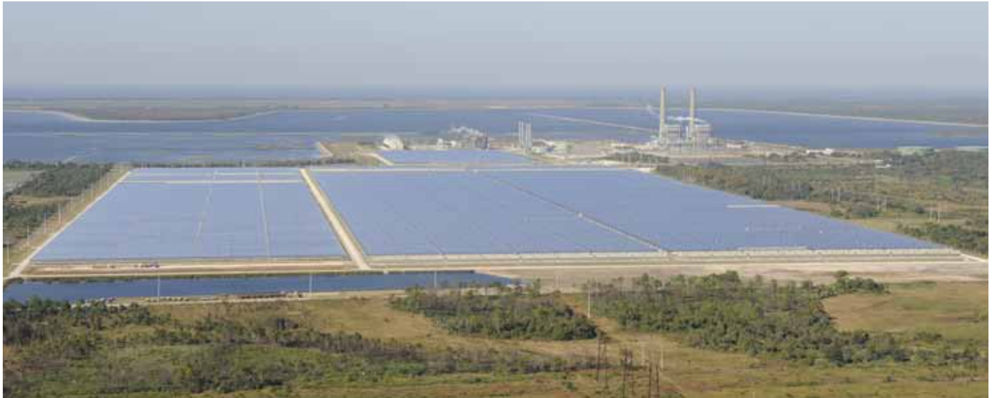
75-MW Martin Solar Plant near Indiantown, Florida
