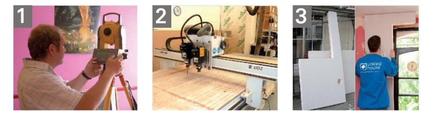
United House – UK: System for the application of internal insulation with minimum effort, low mess and minimal impact on the user, fast and economical. **Three-part process**.
